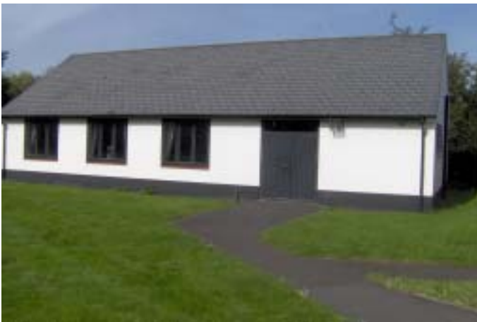
The Parish Hall on St Peter's Site
